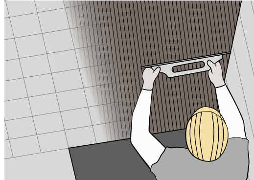
Spread adhesive on the existing substrate
