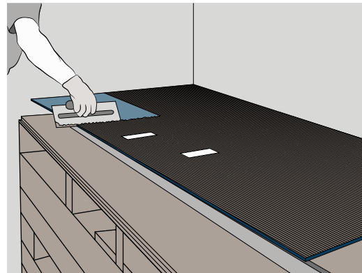
Spread adhesive on the back of the slab
