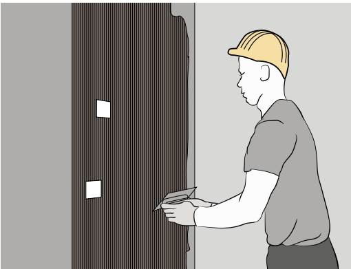
Spread adhesive on plaster
