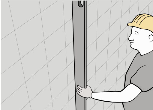
Check planarity of the existing substrate
